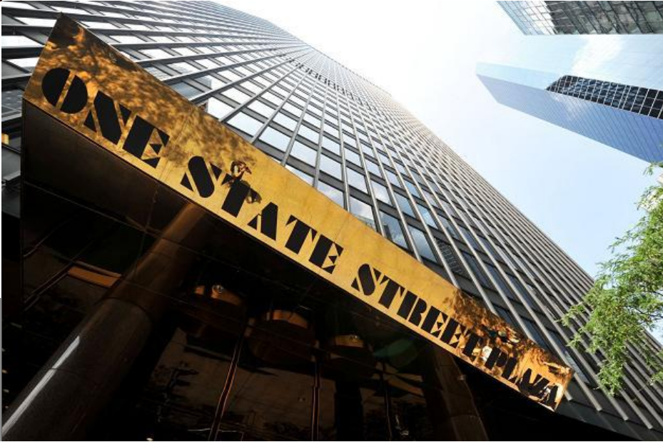
Microbial Assessment One State Street Plaza Client: GEI Consultant
